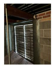
Choir loft attic: Above the choir loft are two old ventilation panels that need to be sealed off and an access door to the roof included in the one of the panels.
